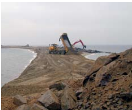
Poplar's progress – closing one of the containment cells
